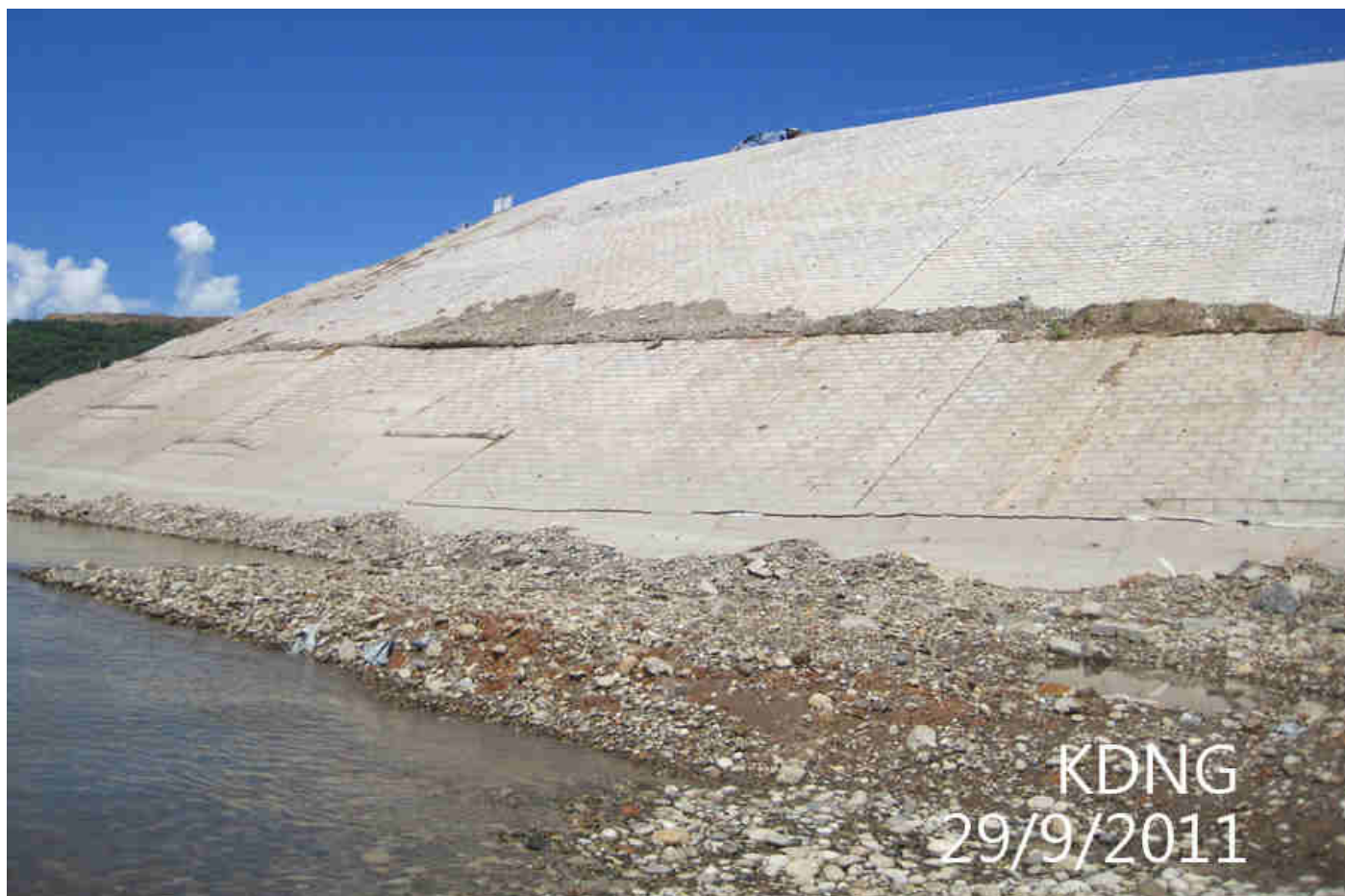
A containment wall downstream of the Myitsone dam site is already cracking, possibly due to poor quality materials or poor construction standards.
