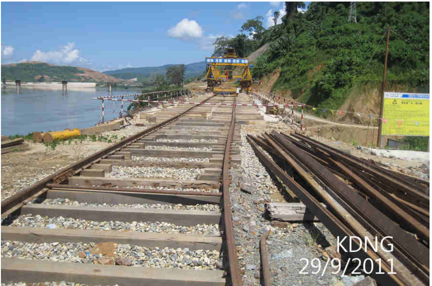
A railway to transport equipment and materials between construction sites at the Myitsone Dam
