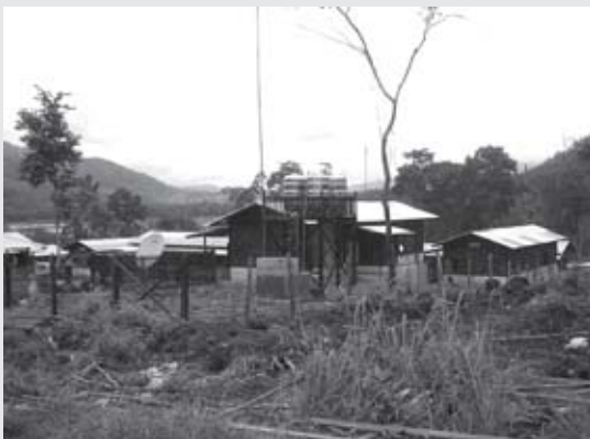
Asia World's base camp at the dam site
